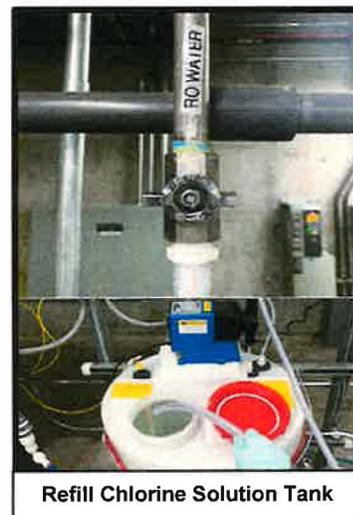
4. While the RO machine is making water, zero the test meter, wait five (5) minutes, then test the free chlorine levels using the approved test kit.
